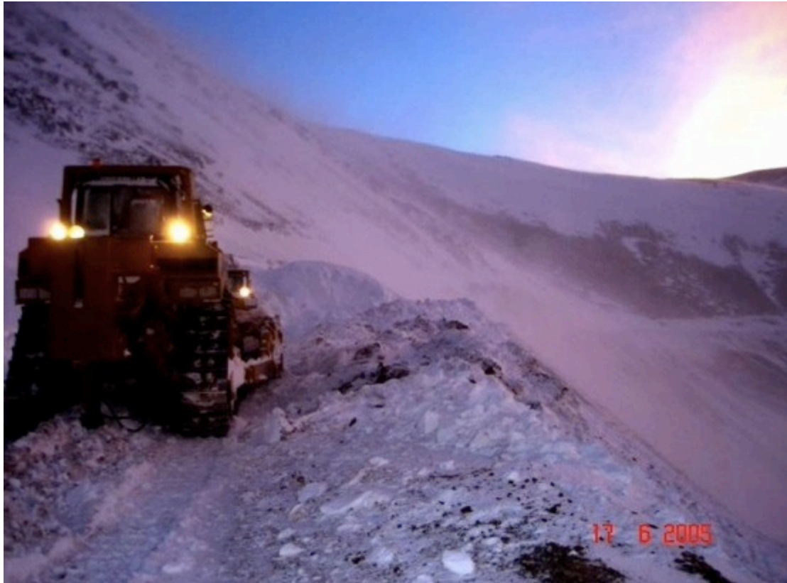
Barrick subcontractor Zlato's bulldozer in 2005 removing ice from Conconta Pass. Source: Zlato
