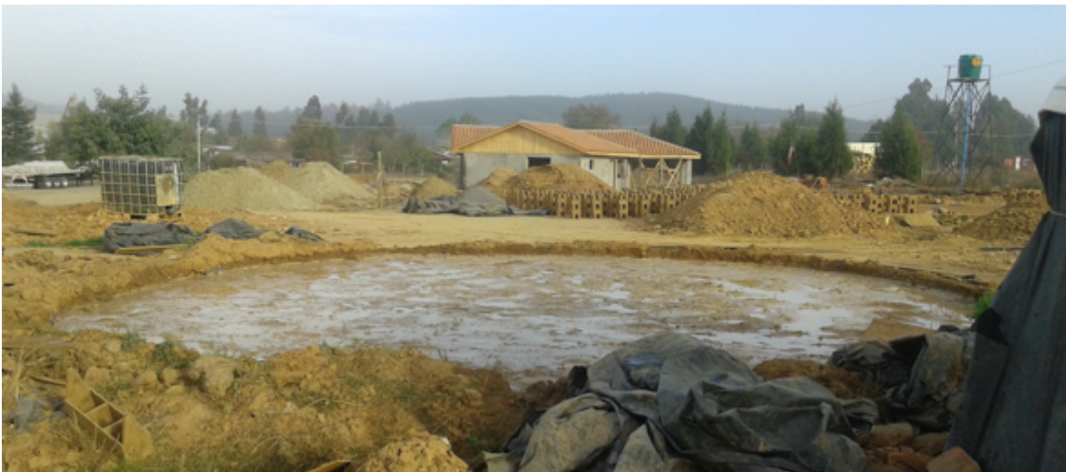
Clay mixing pond adjacent to Traditional Brick Manufacturing site. Cauquenes, Chile
